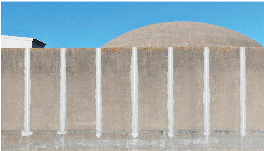
Monitoring of the dike
